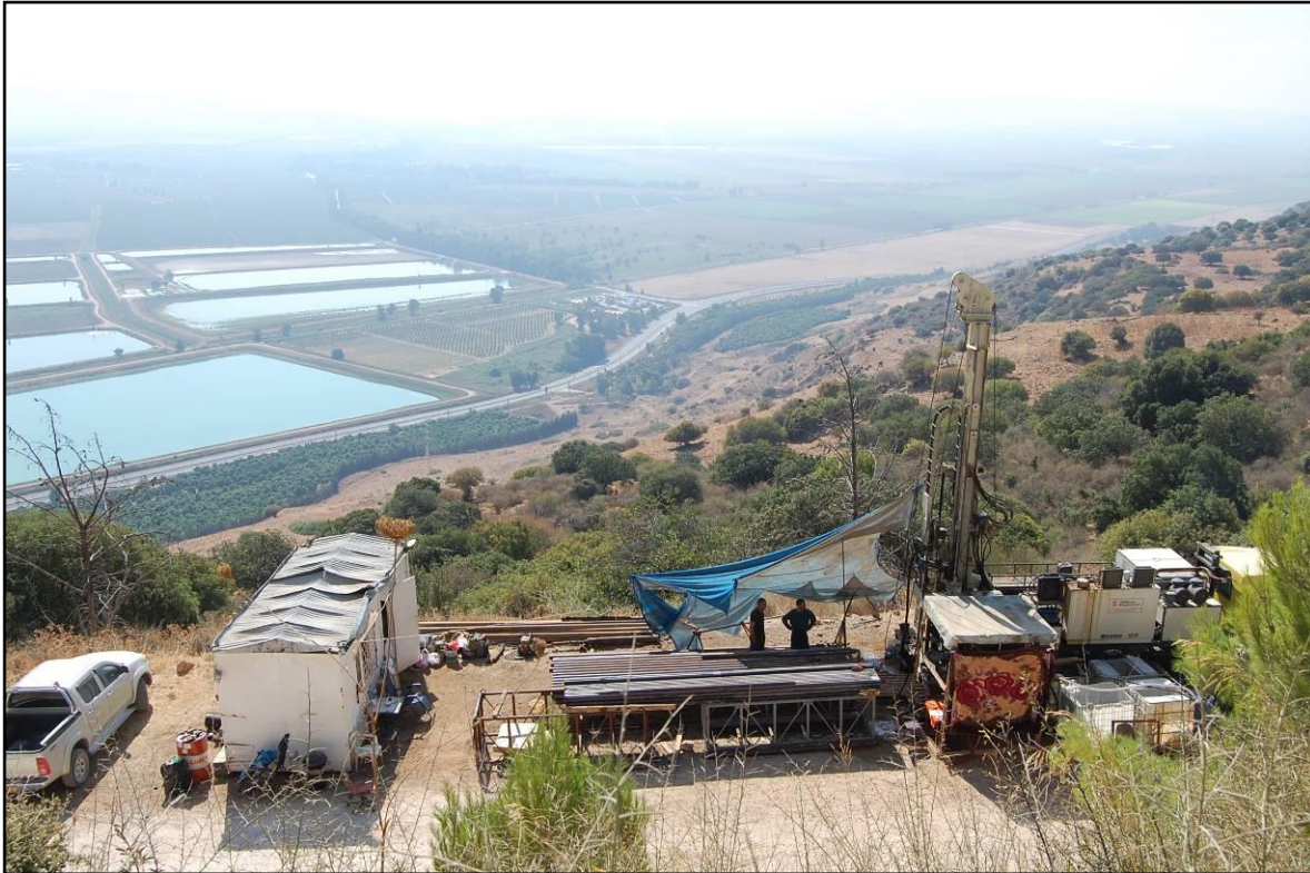
Figure 6: The MNUPH-1 borehole site on the mountainside above the lower reservoir.
